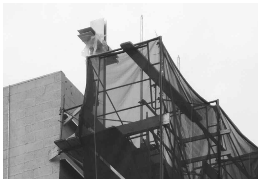
Installation of cross on W83 building
